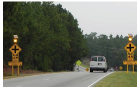
Example of countermeasures on the through approach. Source: South Carolina DOT
