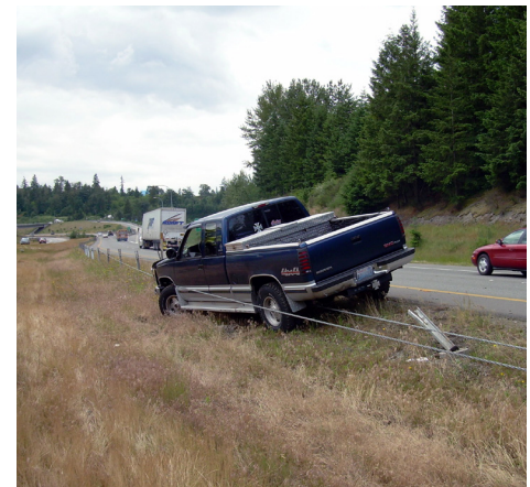
Median cable barrier prevents a potential head-on crash. Source: Washington State DOT
