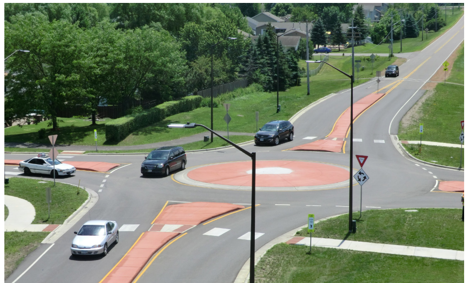
Example of a single-lane roundabout. Source: FHWA
