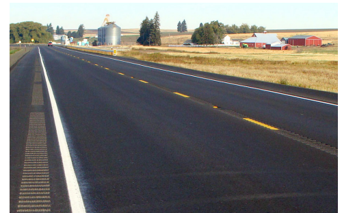
Shoulder rumble strips and center line rumble stripes are installed on this roadway. Source: FHWA
